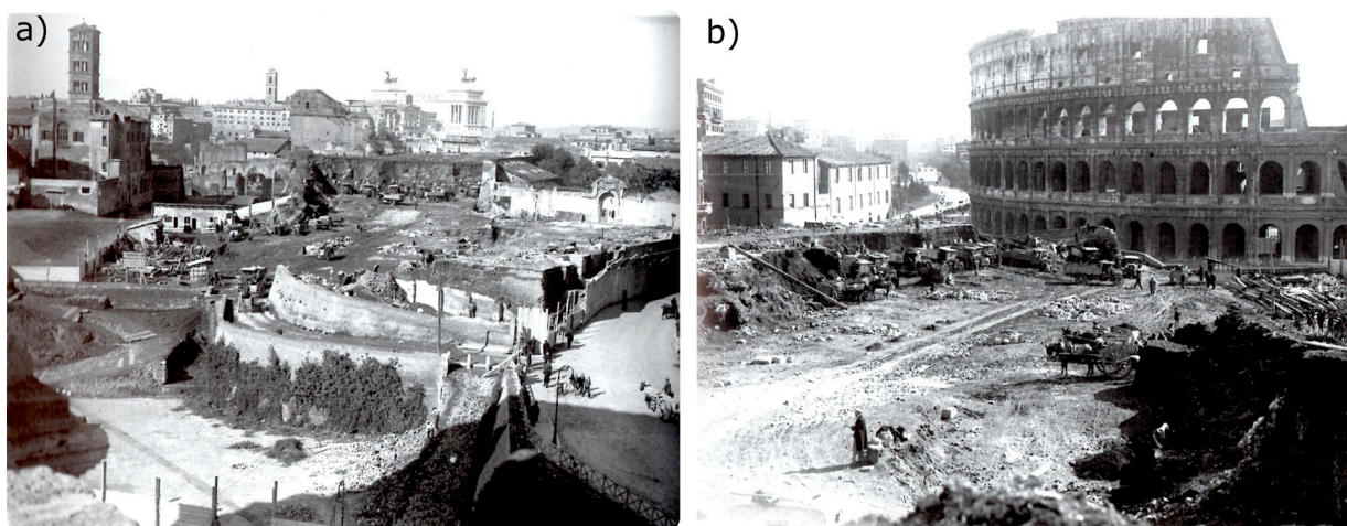
Figure 6. Excavation work on Velia Hill in the 1930s: (a) view from the Colosseum to NW, the Capitoline Hill and the Vittoriano are in the middle background, the Basilica di S. Francesca Romana in the upper left corner of the picture; (b) view from the Basilica di S. Francesca Romana to SE, to the Colosseum.
