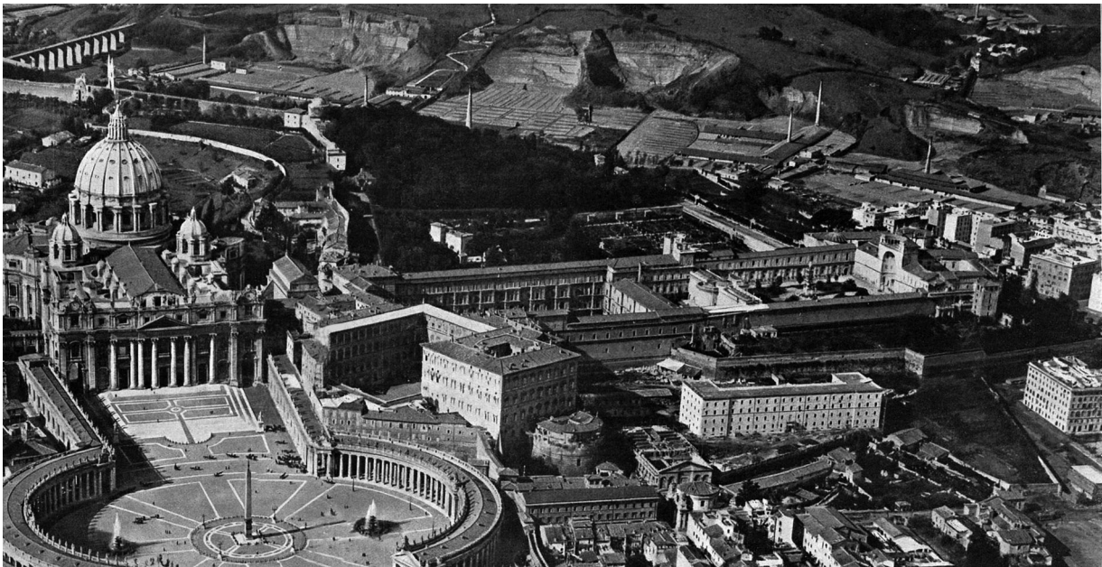
Figure 7. The clay quarries still visible behind the basilica of St. Peter in 1911 were active between the mid-1800s and the 1930s. Clay was used for brick production, which is emphasized by the presence of furnaces whose chimneys are visible in the picture (Insolera, 1985). These quarries have been mapped as abandoned quarries (see the Main Map ).
