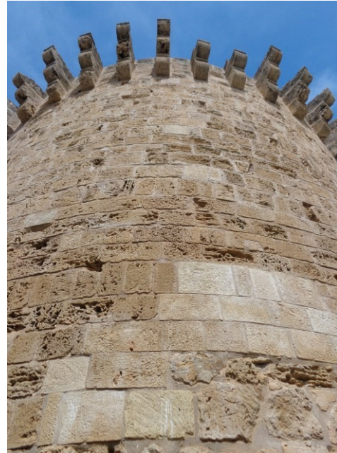
Fig. 4- View of the coronation system of the tower (Camiz, 2018)
