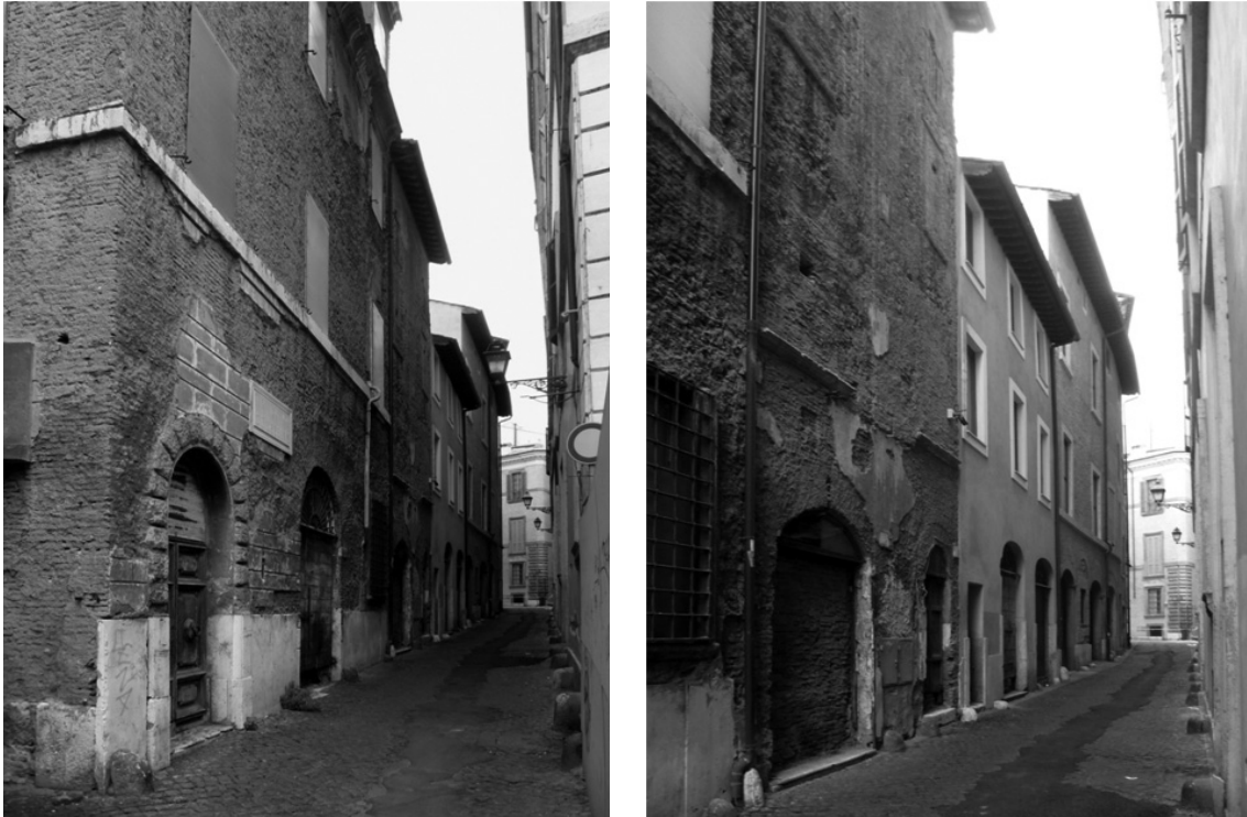
Figure 16-17. Row houses and in linea houses in Via dei Delfini.
