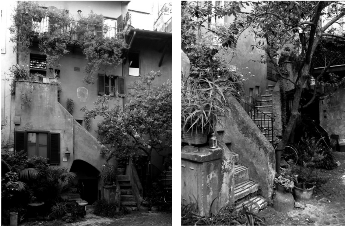
Figure 4-5. Profferlo houses in Arco degli Acetari (courtyard of the via del Pellegrino block).
