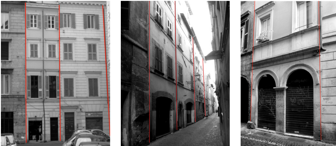
Figure 8-9-10. Row houses in via dei Cappellari. Row houses in via del Pellegrino extensively transformed in the Nineteenth century. It is still possible to recognize the original type with double window and double doors.
