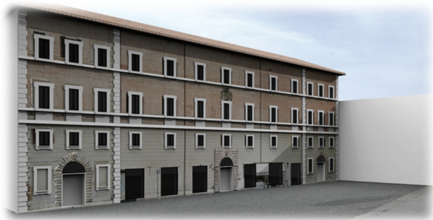
Figure 13. 3D model of Palazzo della Famiglia in Piazza Borghese. The elevation is textured by projecting the equi-rectangular image from the Google panorama.
