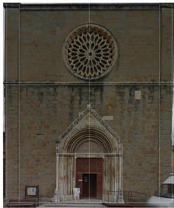
Figure 17. The equi-rectangular image projected from the centre of the panorama on the plane identified, returns an image in true dimension.
