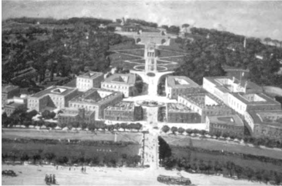
Fig. 20. Perspective of M. Piacentini project for the area of the Regina Coeli prison.
