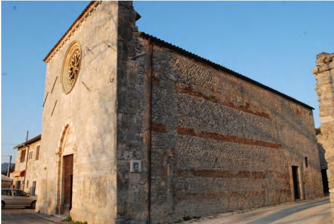
Fig. 68. The opus mixtum of a roman masonry embedded during the construction of the right flank of the church of S. Maria in Pantano in Massa Martana. Photography E. Scopinaro 2016.
