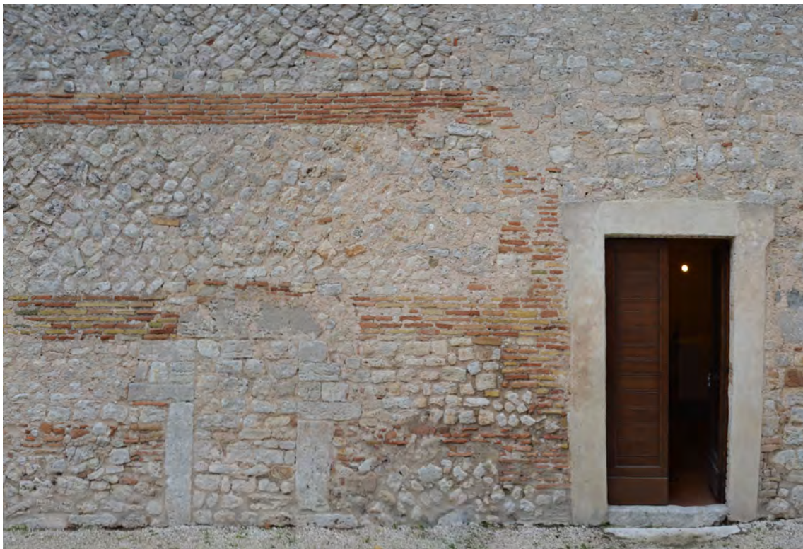
Fig. 73. Masonry of the right flank of the church of S. Maria in Pantano. The down part, built between the 10 th and the 11 th century seems to re-propose the different pose in work in bands according to the Roman example. Photography E. Scopinaro 2017.
