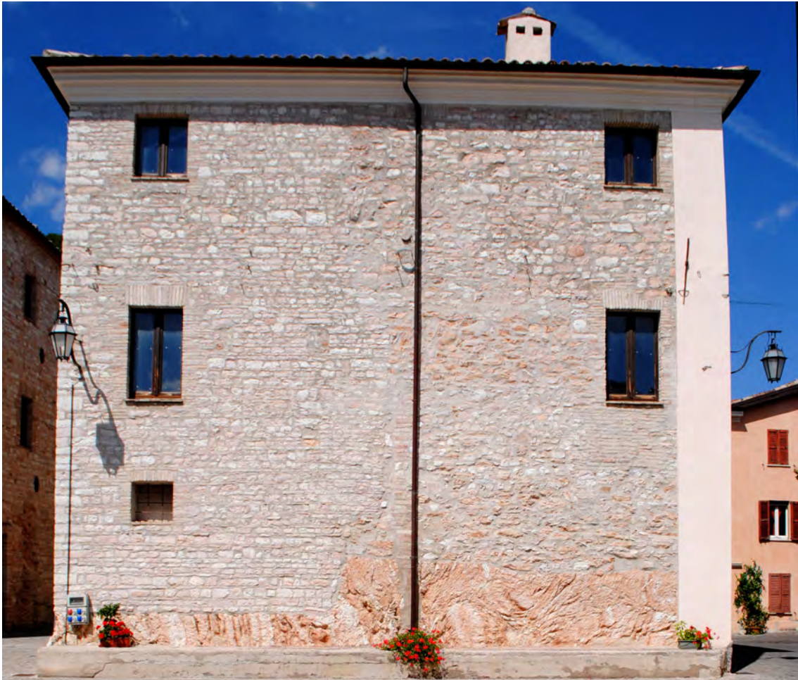
Fig. 52. Buildings in Genga. The construction was built on the natural rock. Photography R. Loreti 2014.
