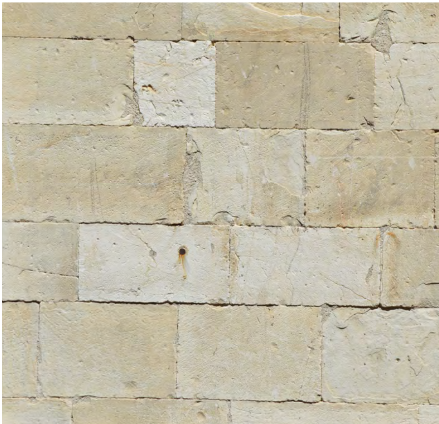
Fig. 81. Detail of the masonry of the right flank of the church of S. Benedetto to Gualdo Tadino. The rocks are smoothed with martellina (bush hammer) and flat chisel on the edges. Photography E. Scopinaro 2016.
