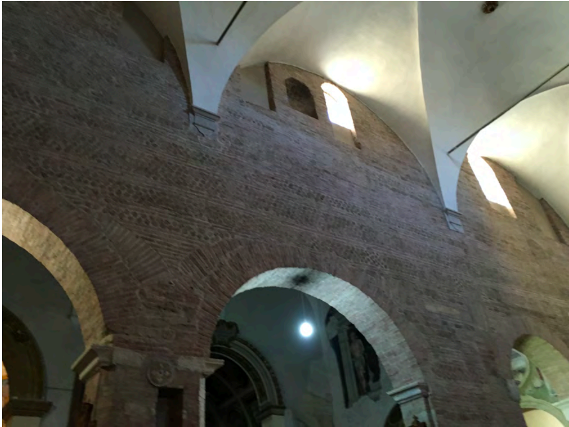
Fig. 72. Masonry in opus mixtum in the church of S. Maria Assunta in Otricoli. Photography L. Barelli 2016.
