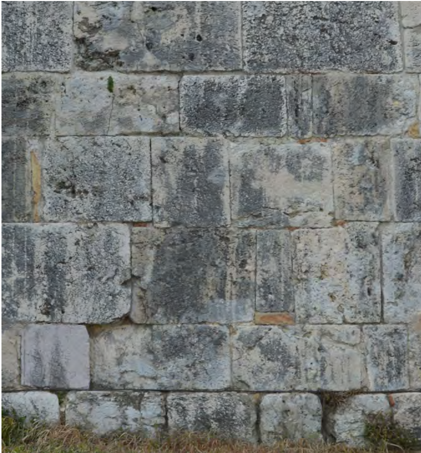
Fig. 50. The church of S. Lorenzo in Ninflis. Detail of masonry made with reused ashlars. Photography E. Scopinaro 2017.
