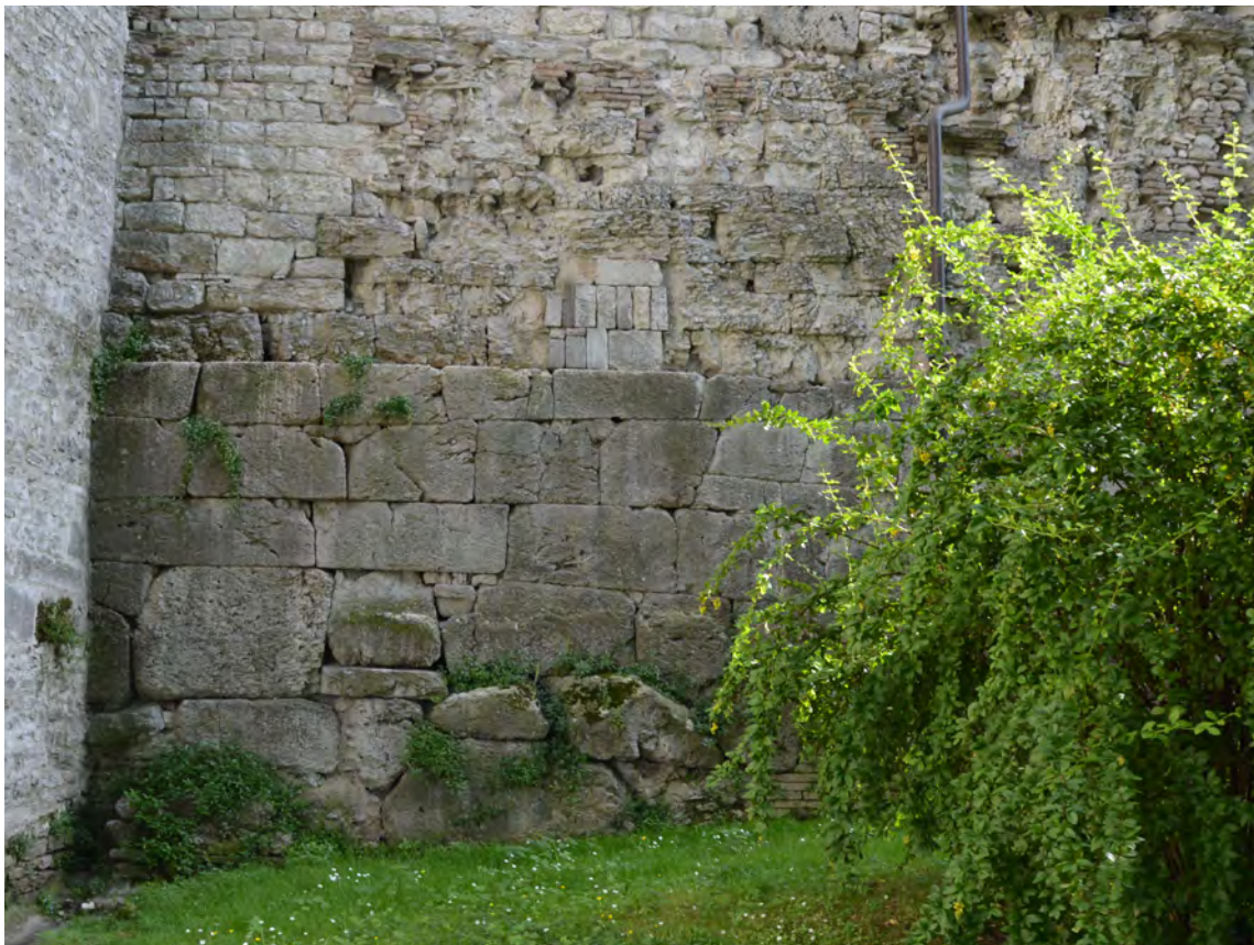
Fig. 61. The spoieto walls. Examples of masonries of first and third manners of opus siliceum and opus quadratum . Photography E. Scopinaro 2016.
