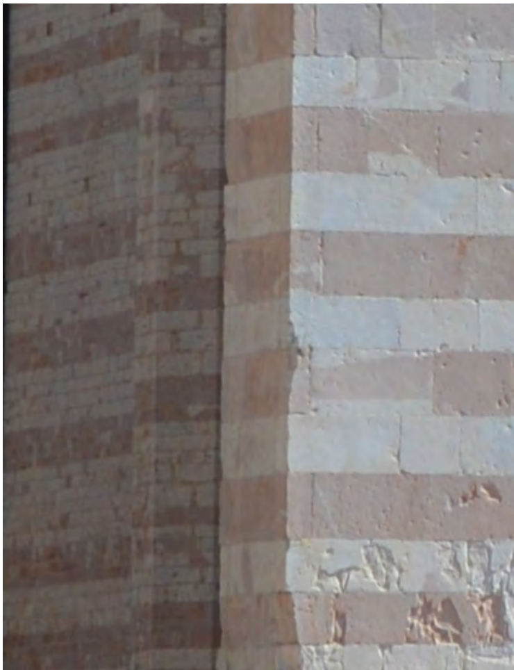
Fig. 96. a. The Church of S. Chiara of Assisi. b. Detail of the connection between the masonry of the side and that of the façade. Photography E. Scopinaro 2017.
