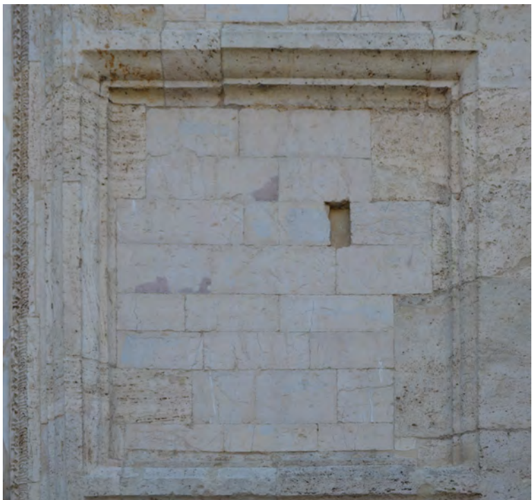
Fig. 107. The facade of the cathedral of S. Rufino in Assisi. Detail of ashlars made of scaglia rossa discoloured. Photography E. Scopinaro 2016.
