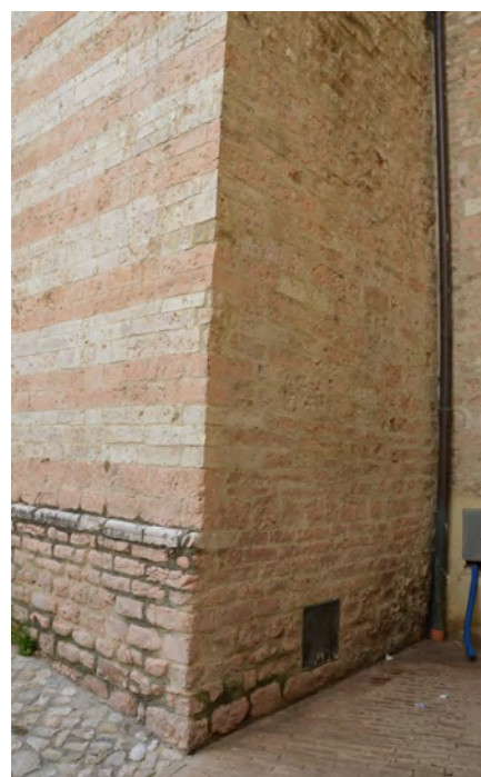
Fig. 89-90. Church of S. Salvatore in Foligno. On the right the detail of the attack of the masonry on the side of the church. Photography E. Scopinaro 2016.
