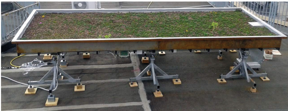
Figure 10: Photo Angle of Prototype with water storage where the state of growth of vegetation clearly highlights the portion of the length is achieved where the accumulation of water, compared to that with inclination greater where, in fact, there is no accumulation of water.
