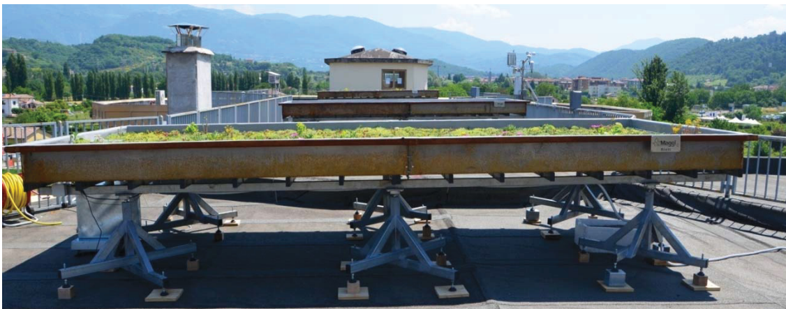
Figure 5: Photo of SOS_UrbanLab: The Test Center. In the foreground the tank containing the prototype of a Green Roof without water storage, the second floor in the bath sample, third floor, the tank containing the prototype of a green cover with water storage
