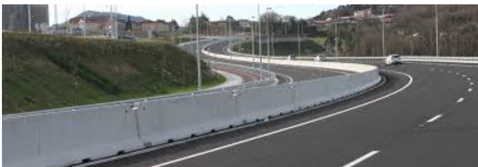
Figure 1. The New Jersey concrete barriers came in Europe between '80s and '90s of the 20th century, after the previous positive experiences in the U.S.
