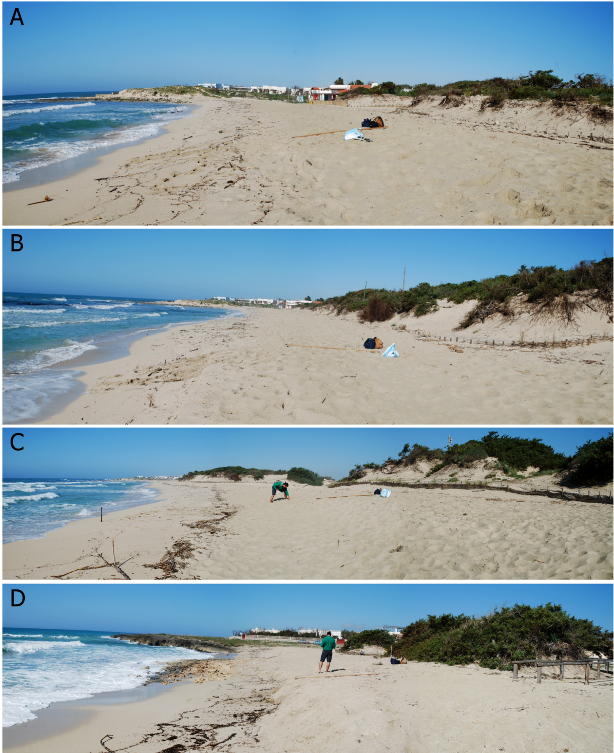
Fig. 13 - Morphological features at the Lido degli Angeli beach. A) Western zone of the beach (photo on profile LA32). B and C) Central zone (profiles LA33-LA34). D) Eastern zone (profile LA36). To note the general degradation of foredunes due to wave-wind erosion and summer recreational activities, the benefits provided by the wood fences, and the calcarenite rocky cup near profile LA36.
