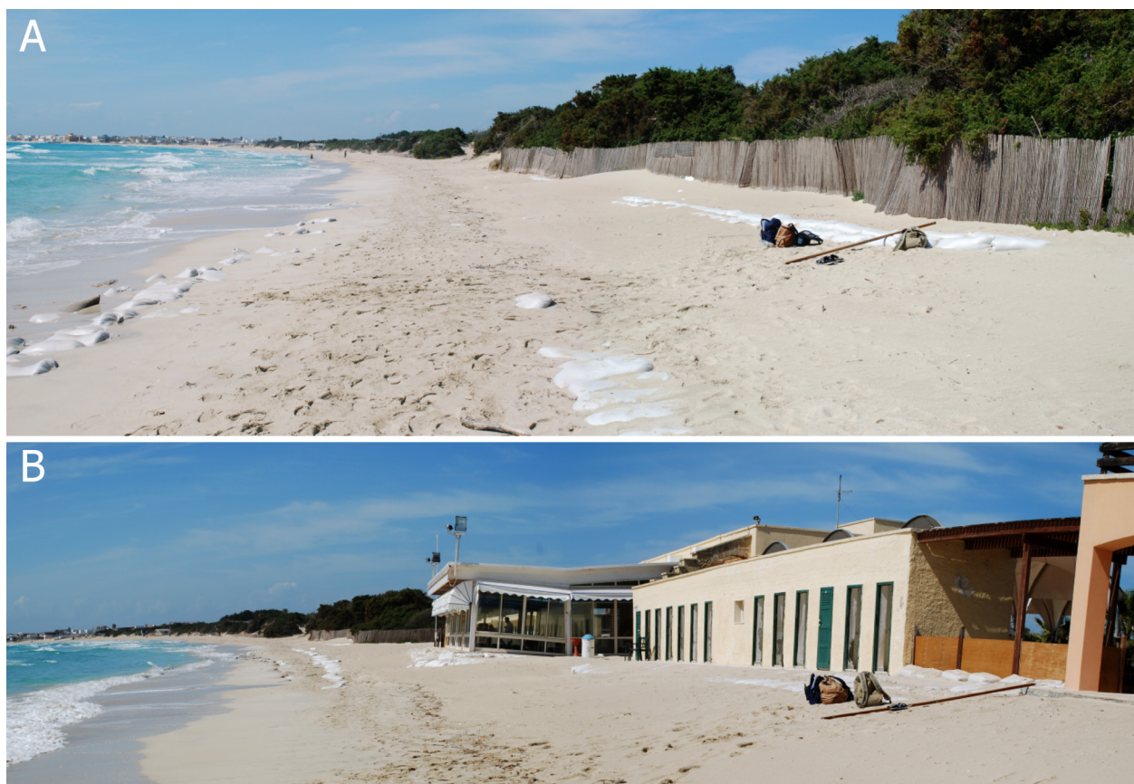
Fig. 17 - A and B) Eastern zone of Torre Lapillo beach near TL 38 and TL39 profiles. Here sandbags and wood fences are used to contrast erosion especially in the Bacino Grande bathhouse, very near to the shore. The benefits of this intervention are local and quite limited.
