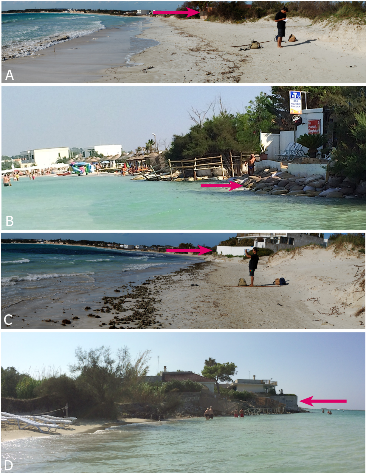
Fig. 16 - Photos collected along the eastern zone of Torre Lapillo beach. A and B) The beach near profile TL45 in April 2010 (A) and August 2016 (B). Note the disappearance of the beach in this time-interval, and the sandbags used to protect the beach resort (see red arrow) from waves. C and D) The easternmost beach portion at the two flanks of the house near to the shore (see red arrow) in April 2010 (C) and in August 2016 (D).
