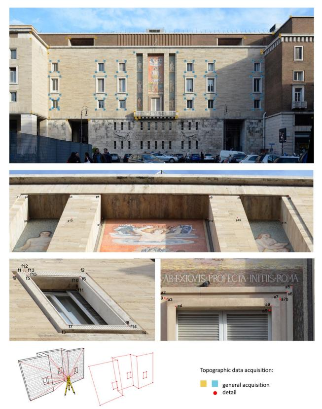
Fig. 2: INPS building: topographic and photographic surveying
