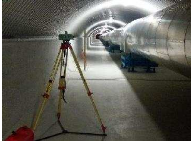
Figure 4: DNA03 station in the Tunnel.
