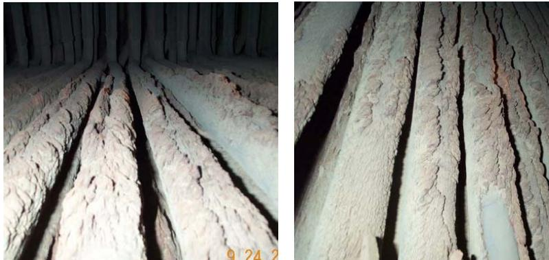
Figure 1.1 – Deposits accumulated on heat exchanger tubes [3].
