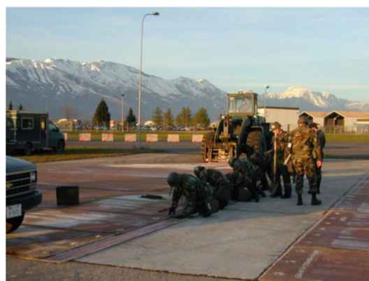
Figure 1. Anchoring the fiberglass mat.
