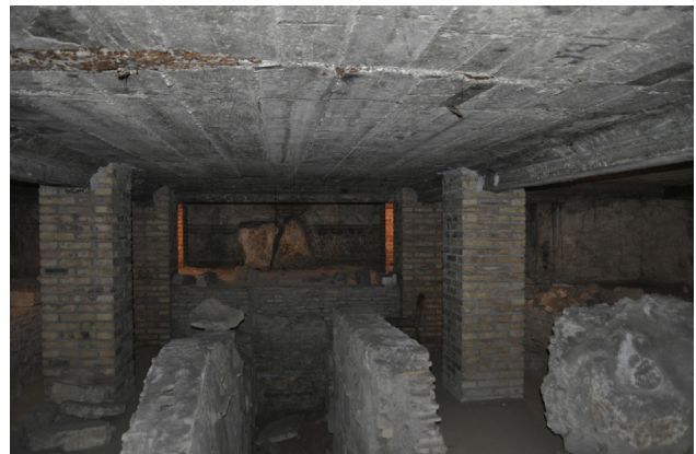
Fig. 5. San Saba Oratory. General view of the building towards the apse.
