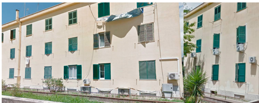
Fig. 7. Chimney and external air conditioning terminals.
