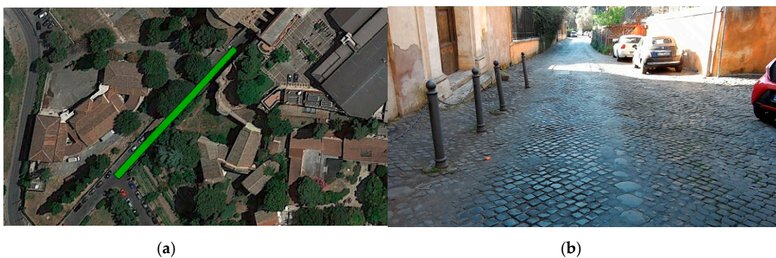
Figure 6. Sampietrini pavement Section 06: (a) top-down; (b) street views.
