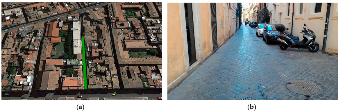
Figure 5. Sampietrini pavement Section 01: (a) top-down; (b) street views.
