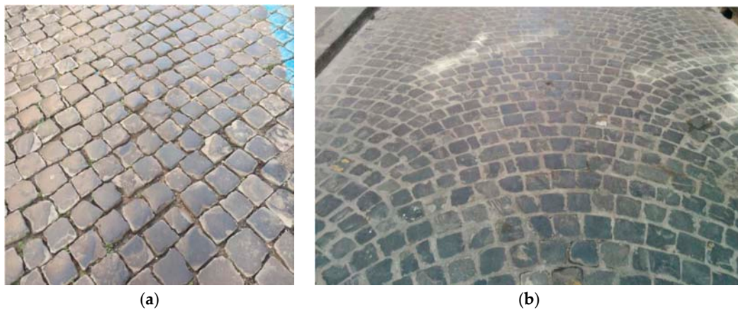
Figure 2. Geometric patterns: (a) herringbone at 45°; (b) arc.
