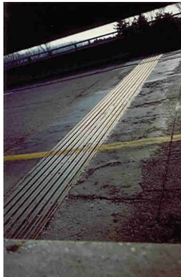
Figure 4. Pavement condition of the area surrounding the BEJ.
