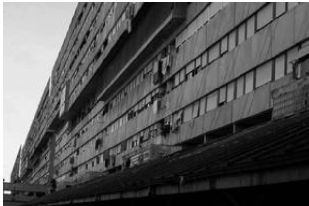
Figure 4. Corviale building, Rome
