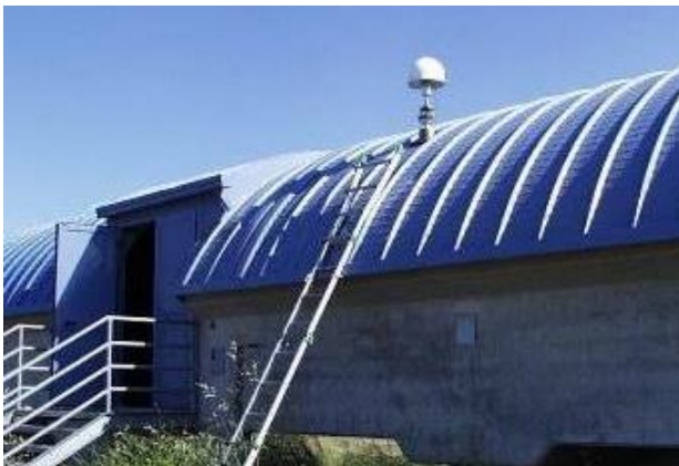
Figure 3: GNSS antenna mounted on the tunnel.
