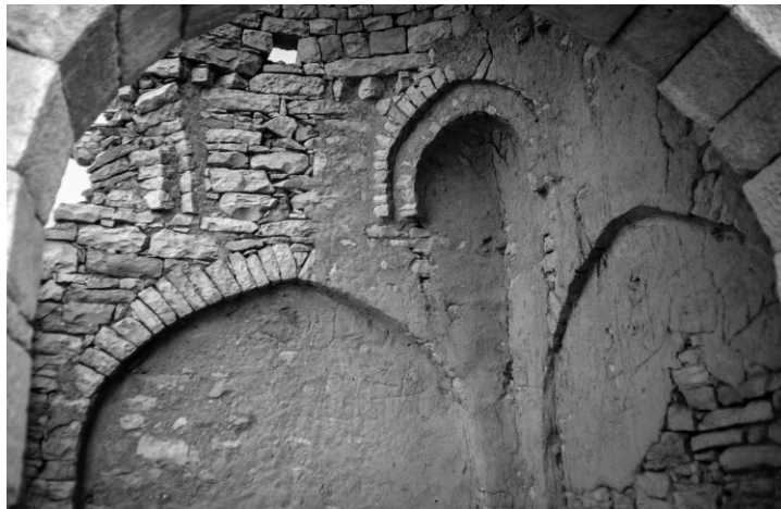
Fig. 6 - Barāqish. The chahār ṭāq mausoleum: the interior, showing a squinch and the lowest rings of the dome (© M.V. Fontana 1992).
