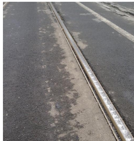
Figure 1. Corrugated rail R, relating a straight section of the right track of a bidirectional line.
