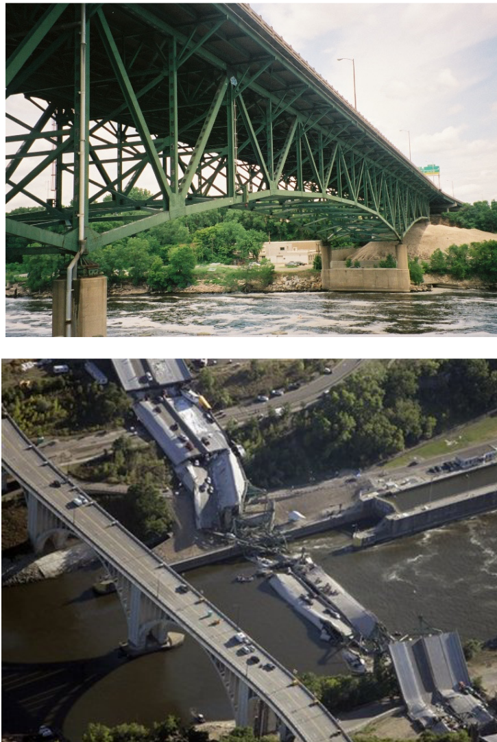
Figure 1-2 - I-35W Collapse - August 1, 2007
