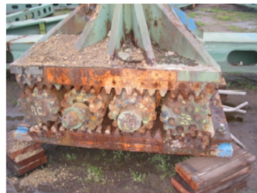
Figure 8-15 - a) 2003 URS photo of Pier 6W bearing U8 (WJE); b) Re-assembled Pier 6 bearing
