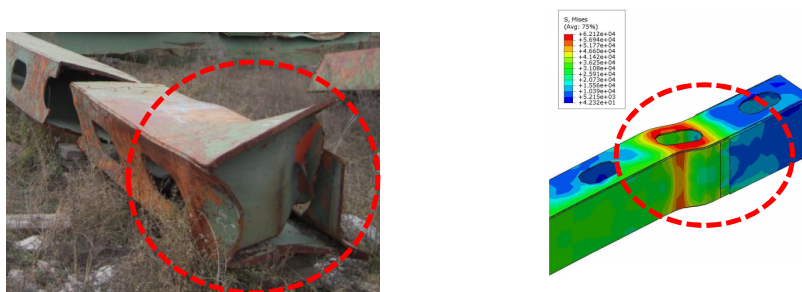
Figure 10-24 - View of the South West Side member L9W-L11W
