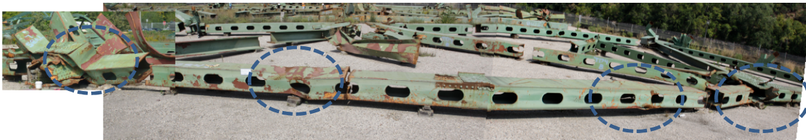
Figure 10-20 - View of the North West Side member L9'W -L11'W
