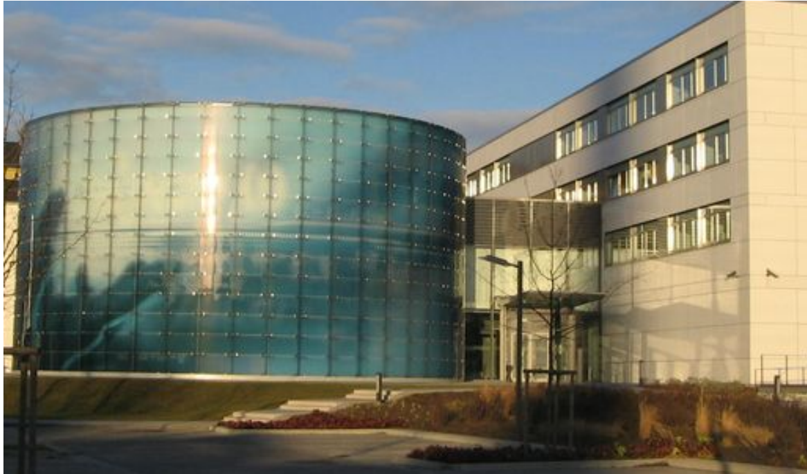
Fig. 13: external view of the ED.
