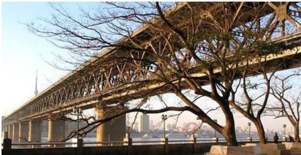
Figure 4.8. Bridge with X diagonal, First Whhan Bridge in China. (Wikipedia)
