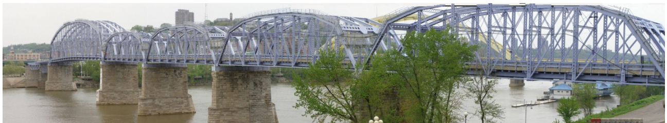
Figure 4.7. Newport Southbank Bridge in Ohio. (Wikipedia)
