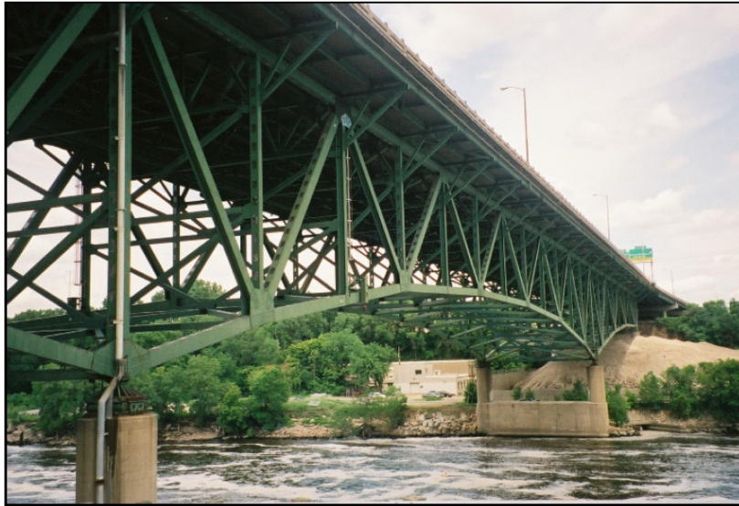
Figure 5.1. Example of truss bridge with gusset plates. (Photo by NTSB Report).
