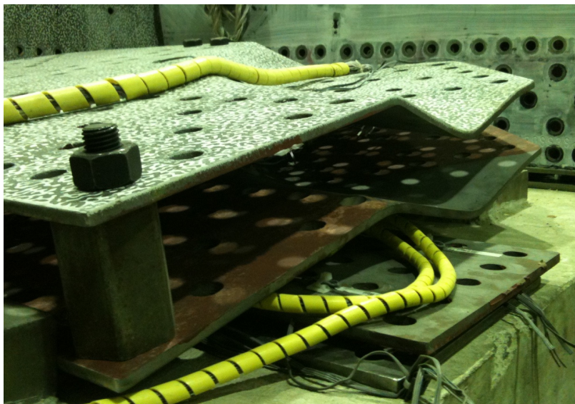
Figure C.4. Results of these tests, buckling of the gusset plates.
