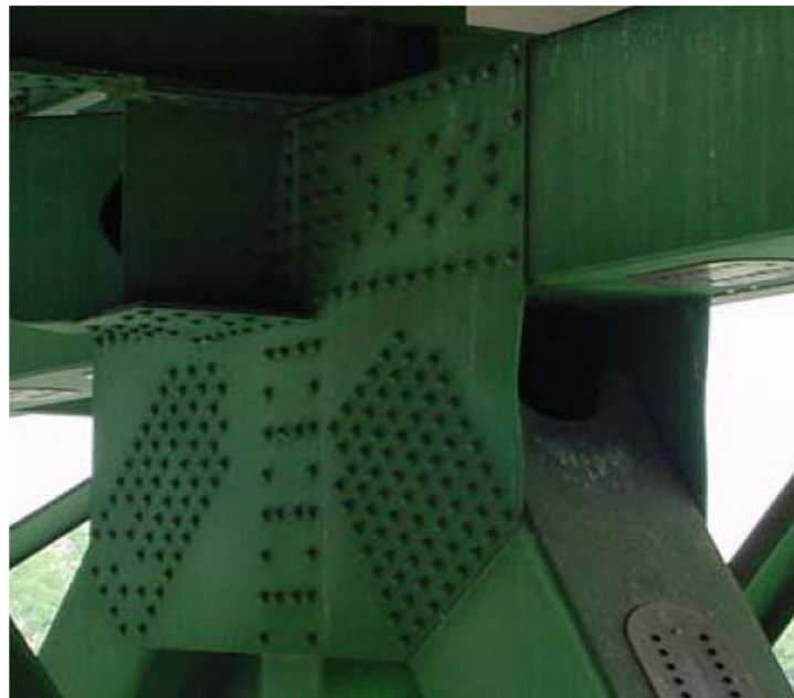
Figure 9.25. Picture of U10 W connection taken on June 2003, [NTSB, 2008].
