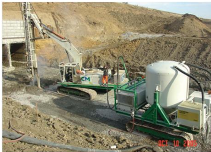
Figura 1.9 - Trattamento dry mixing (Bohem, 2012).
