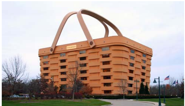
Longaberger bldg, Newark, Ohio, 1997
