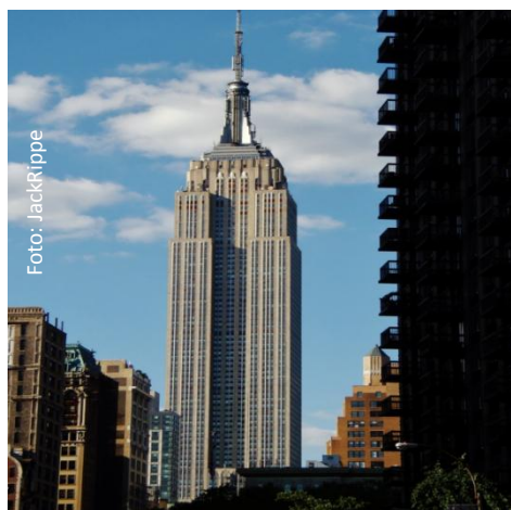
Fig.191. Empire State Building
