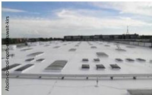
Fig. 211. Carrefour, copertura cool roof
