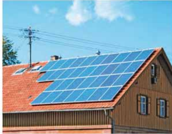
Figure 8.6. Domestic photovoltaic power generating system [204].
