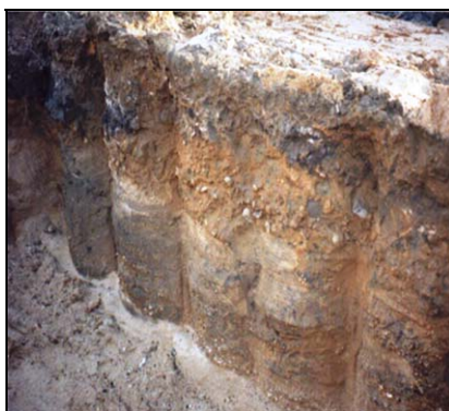
Figura 2.3 – Barriera in deep mixing.
