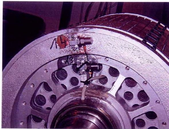
Fig.3.A.2. Sensor installation on end-ring and stack. (Source: Muller-BBM).
