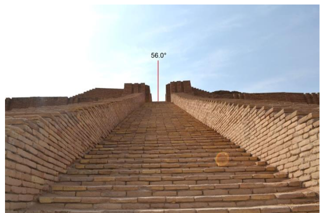
Figura 5: Measurement of the frontal staircase of the Ziqqurat (photo by the authors).
