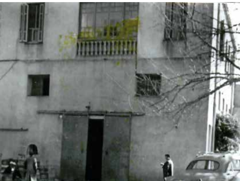
4. Wine cellar of the company Brignone in Grombalia.
