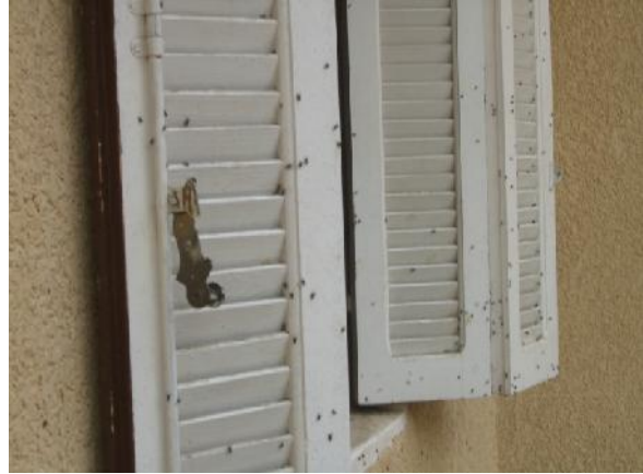
Picture 21: Flies on the school shutters
