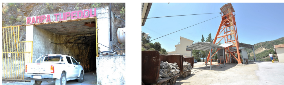
Figure 5.8: The two main access of the Sos Enattos mine: on the left the tunnel rampa Tupeddu , on the right the vertical shaft.
