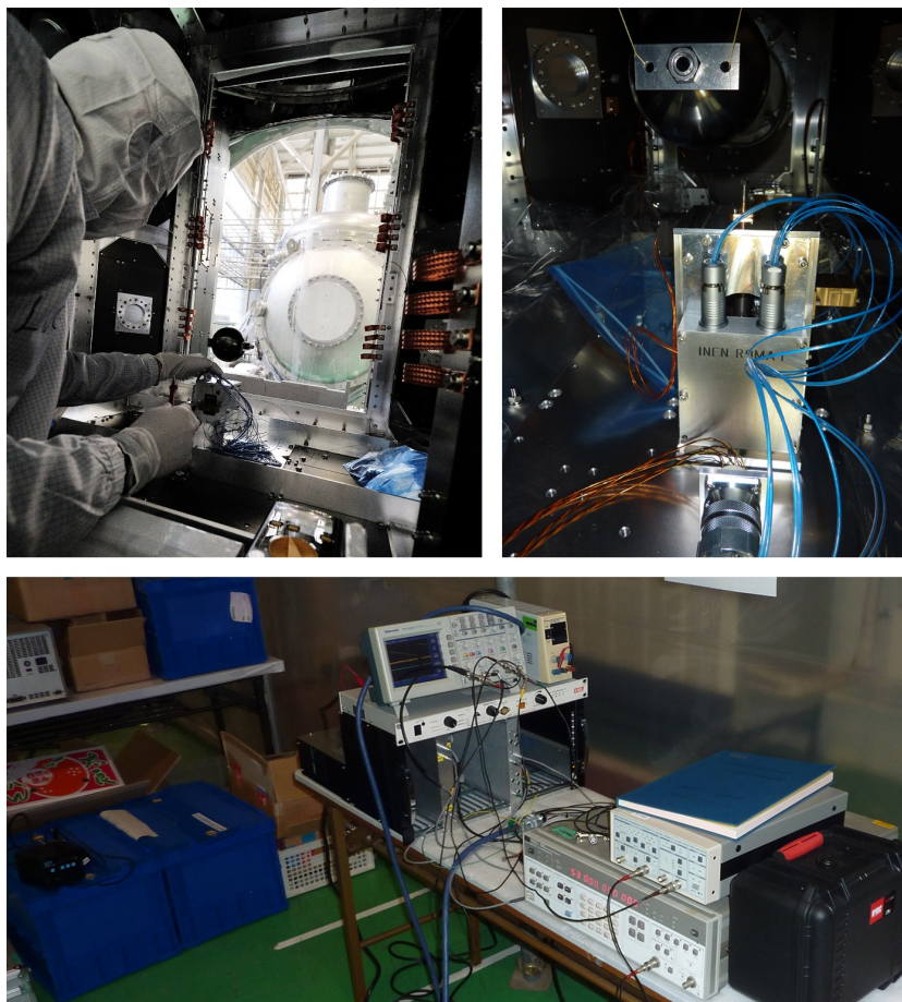
Figure 6.33: Installation of the cryogenic vertical accelerometer into the cryostat #2 of KAGRA. From left, clockwise: installation phase in clean-room environment; the accelerometer fixed to the support platform on the radiation shield and cabled to feedthrough cables; external instrumentation setup.
