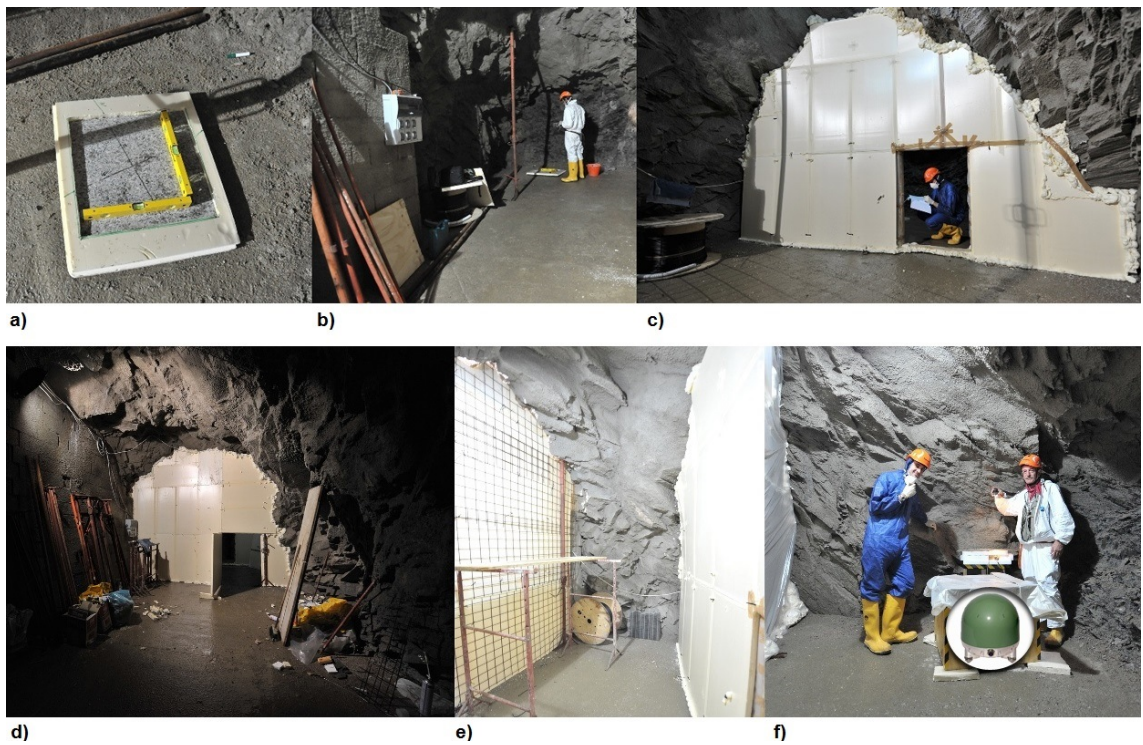
Figure 5.12: Insulation and instrumentation of station -2 in Sos Enattos, from top-left to bottom-right: a) the granite plinth, leveled and cemented on the bedrock; b) the cave before the insulation; c) the first insulation wall, made of polyurethane and mineral-wool layers; d) the second insulation wall, also made of polyurethane; e) the outer room between the two insulation walls, before the installation of the DAQ and power instrumentation; f) installation of seismometer Trillium 240 (indicated by the circle), placed on the plinth, inside the inner room: the sensor is enclosed in a thermal shield plus an external insulation box.
