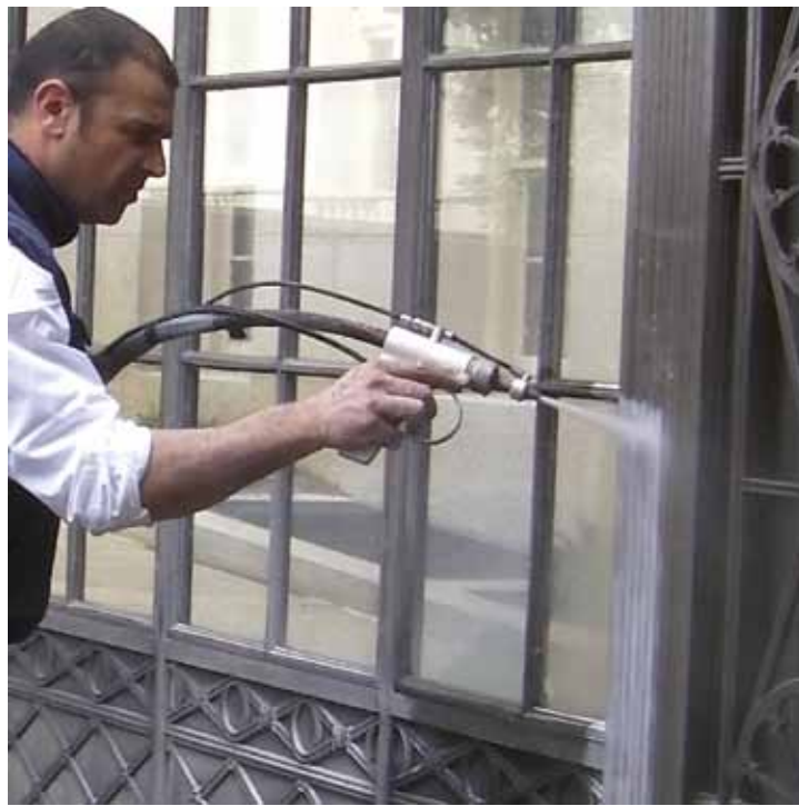
Fig. 8. The HELIX helical vortex technology for aero-abrasive cleaning.
