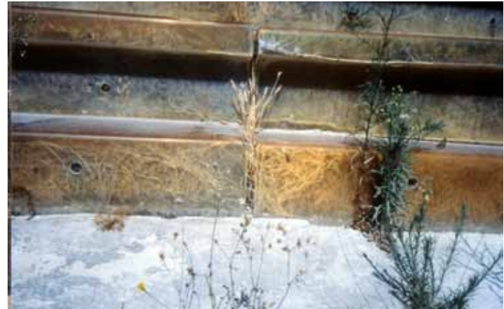
Fig. 2. Proliferation of plants inside the plastic roof system.
