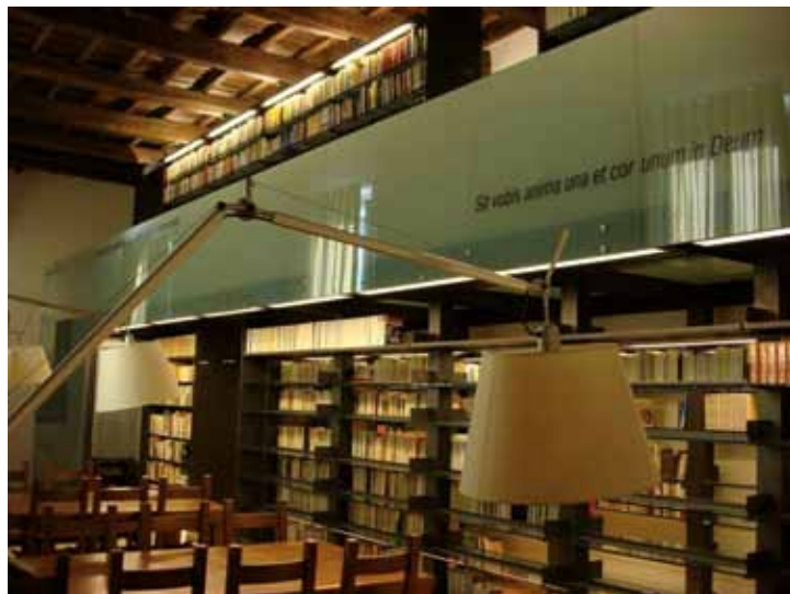
Fig. 3. Ss. Quattro Coronati, Rome – The structure of the consolidation of the wood slab is also the frame of the library and integrates electrical and lighting while the heating is radiant underfloor.
