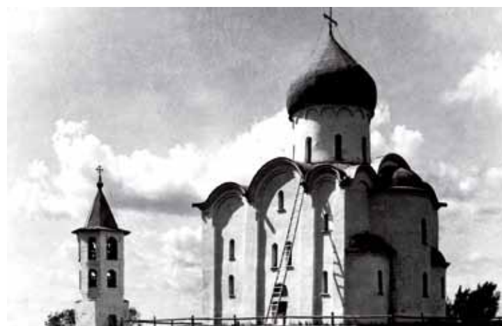
Fig. 6. Novgorod. Church of the Savior on the Nereditsa after the restoration in 1904.
