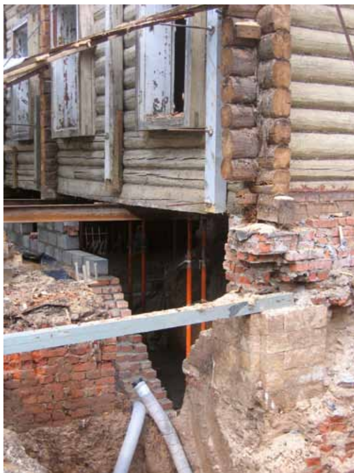
Fig. 5. Restoration of the foundation of the estate of Malvinskoe (Otrada). Photos 2009.
