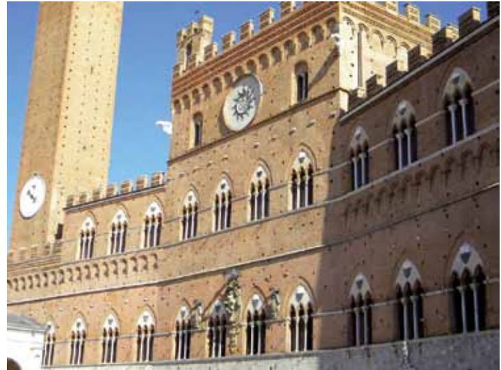
Fig. 3. Siena (Italy). Town hall. The medieval building was elevated in 1680-81.
