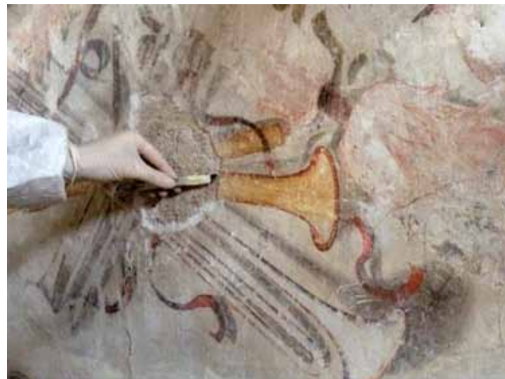
Fig.6. Restoration of painted decorations discovered during the works.
