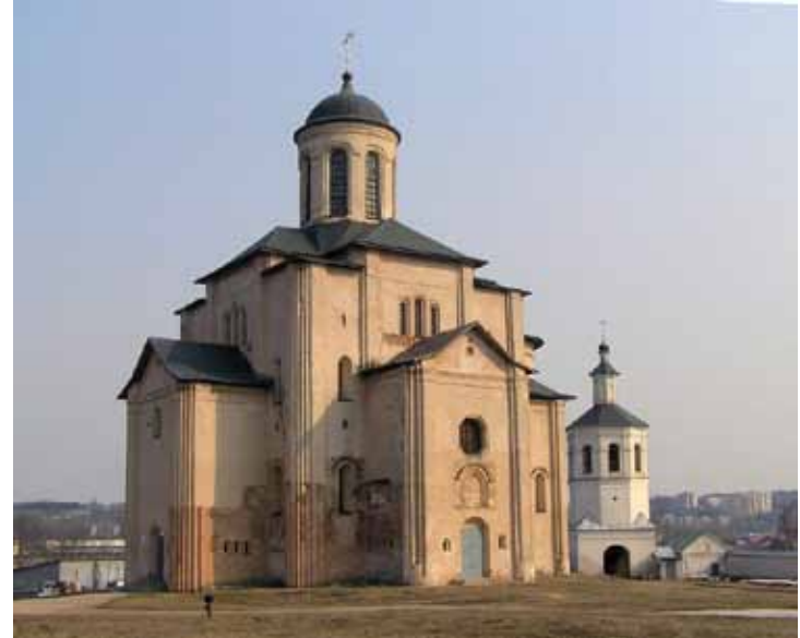
Fig. 16. Smolensk. The Church of Michael the Archangel (the 12th century). Restored by S. Pod'yapolskiy, T. Kameneva. 1979 - the 1990ies.
