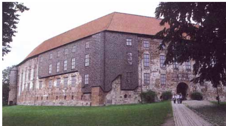
Fig. 3. Koldinghus (Denmark), the castle restored (archh. Inga e Johannes Exner).
