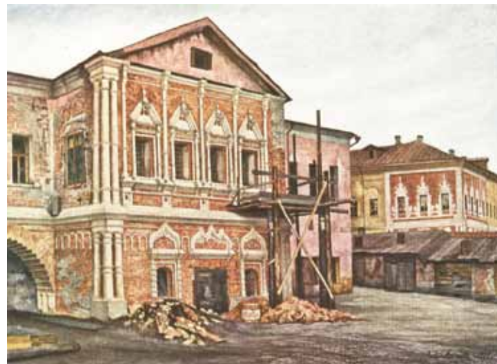
Fig. 8. Moscow. V. Golitsyn's Chamber (end of the 17th century) The view in the course of restoration in the 1920ies. Artist V. Kolenda, 1930.
