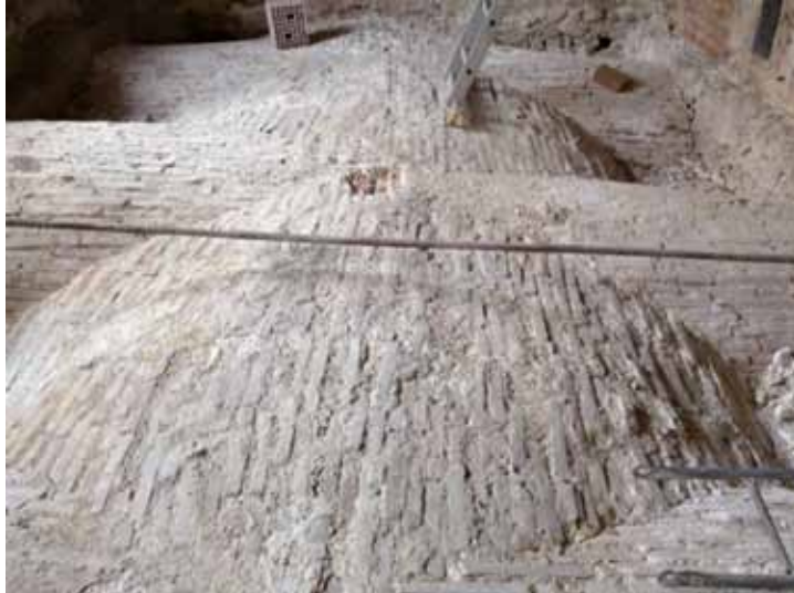
Fig. 3. The double cross vaults of the portico.
