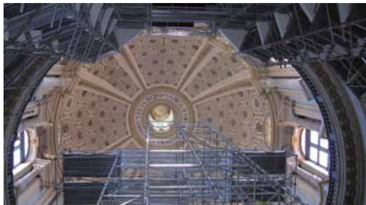
Fig. 3. View of the Superga Basilica dome's with scaffolding.
