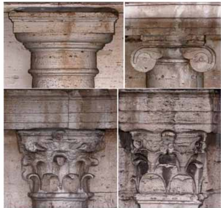
Fig. 9. Coliseum, Rome (Italy): Façade North: details of the capitals (I, II, III, IV order) (Ph. B5 srl).
