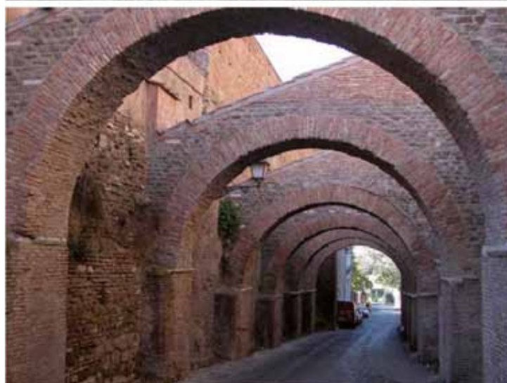
Figs. 1-2. Two historical examples of wall consolidation: above are the medieval buttresses of the Basilica of San Giovanni e Paolo in Rome and below the ancient.
