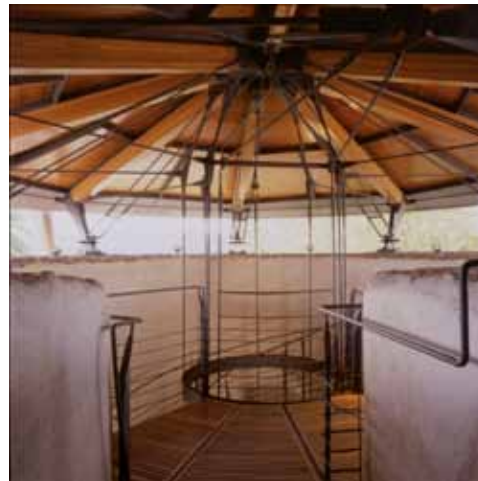
Fig. 8. Gallese (VT): the wooden and steel structural system of the roof of the tower.
