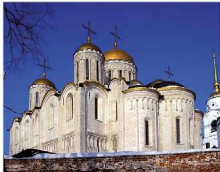
Fig. 3. Vladimir. Cathedral of the Dormition. View after the restoration. Today.
