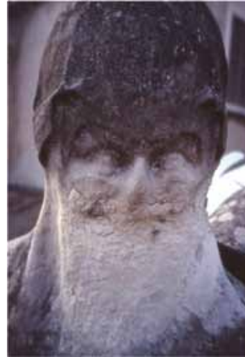
Fig. 7. The advanced state of degradation of the copy of Cangrande's statue.
