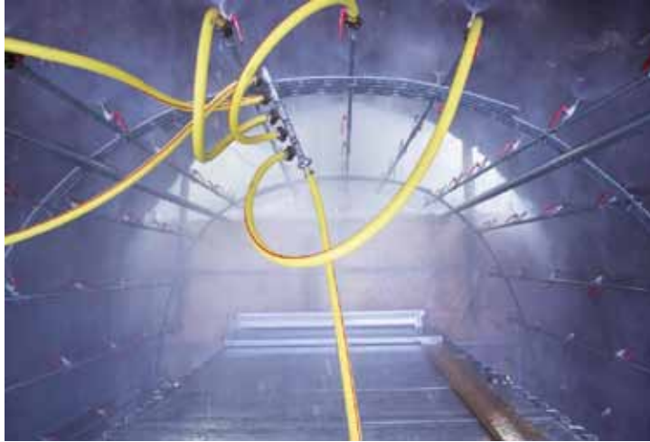
Fig. 5. Coliseum, Rome (Italy): Water nebulization system adapted to shapes and volumes (ph. Tod's).
