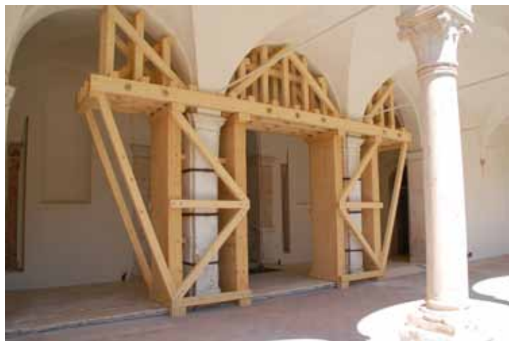
Fig. 4. The provisional strengthening structure of the entrance columns and arches.
