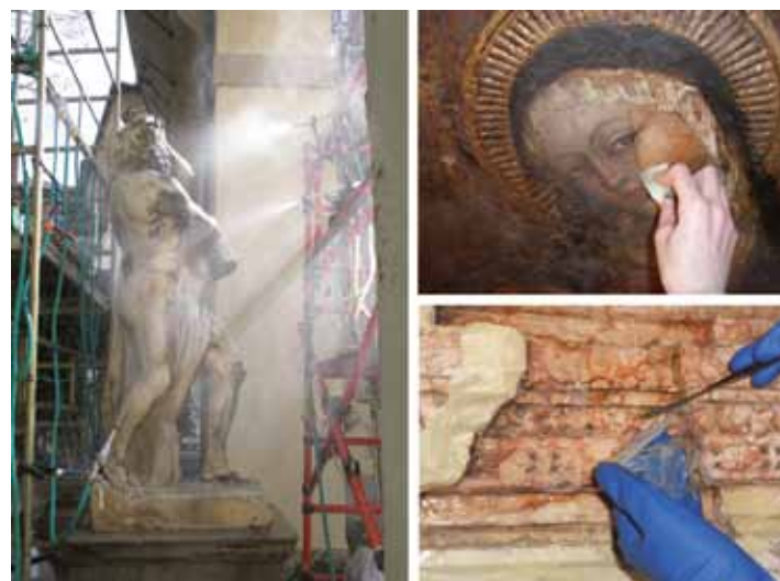
Fig. 6. Use of alternative and low environmental impact substances in the cleaning phases.
