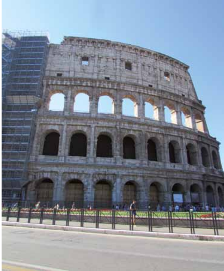
Fig. 7. Coliseum, Rome (Italy): The already restored fornices (ph. B5 srl).
