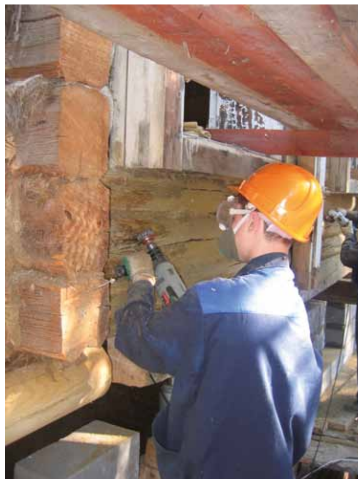
Fig. 6. Restoration of the wooden frame of the estate of Malvinskoe (Otrada). Photo 2009.
