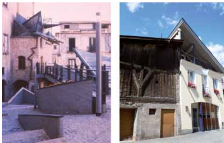
Fig. 5. Meeting between “old and new”, compatibility issues: a) Cosenza, insertion of contemporary elements, b) Vipiteno (Bolzano), juxtaposition of diversified parts.
