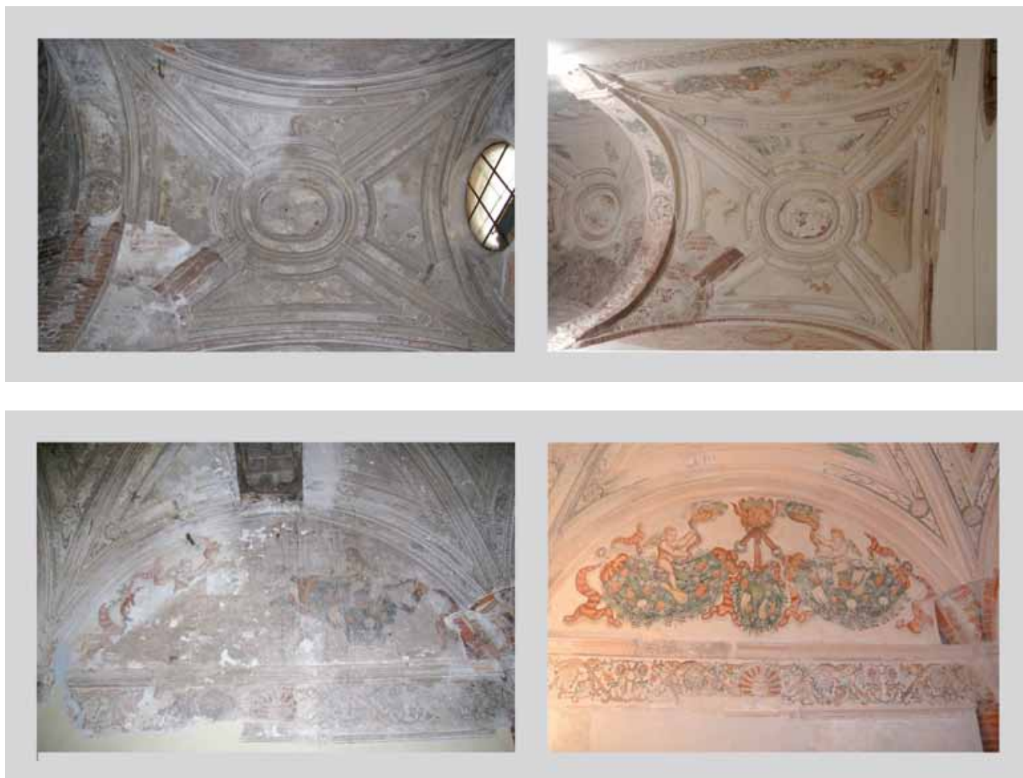
Figs. 5-6. The restoration of decorated surfaces. Detail of a decorated vault before and after the conservative intervention. Detail of a fresco before and after the conservative intervention.
