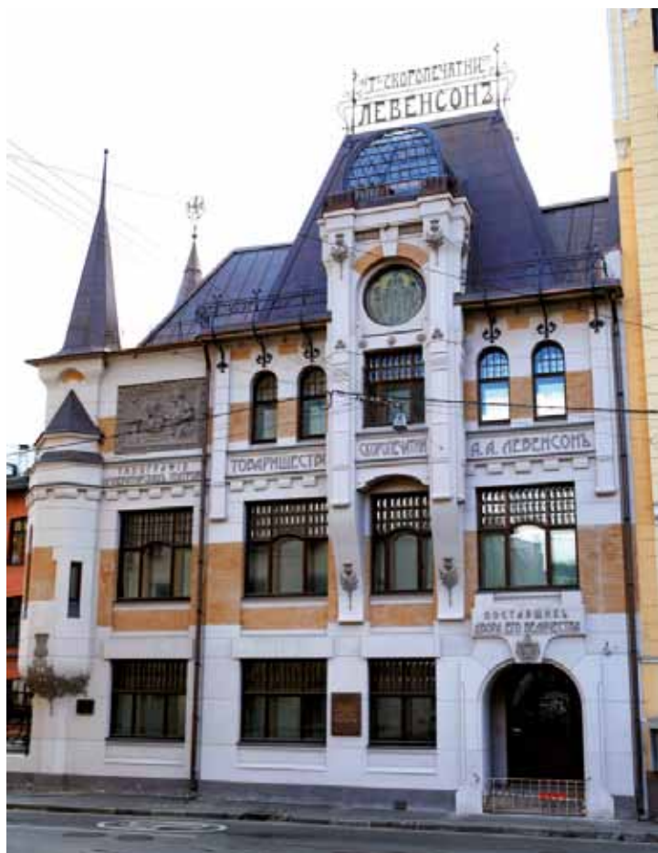
Fig. 7. Object of cultural heritage of federal importance. The Printing House building of A. Levenson, 1900, architect F. Shekhtel. Photo facade of Trekhprudny Lane after the restoration. Authors: Konev Sergey - Scientific adviser; Koneva Ekaterina- Chief architect of the project; Shvechihin P.I. - designer; Tankova N.L. - technologist.
