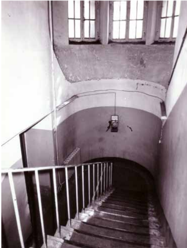
Fig. 8. The interior of service stairs of Levenson's Printing House. Photo 1991.
