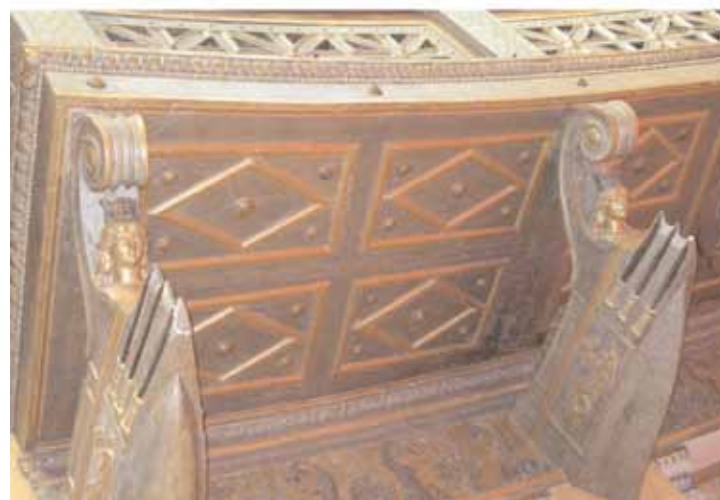
Fig. 5. Acquario Romano. The design of air conditioning systems fit in the old plant passes through integration into the structures of '30 and later.
