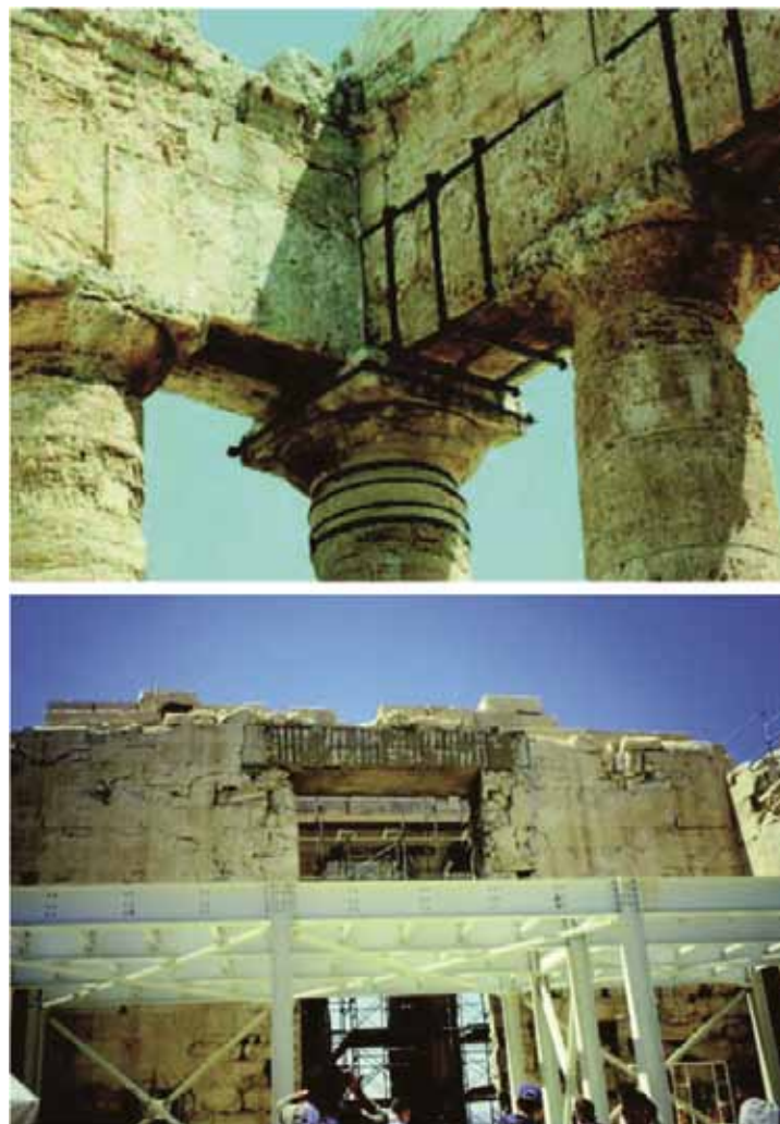
Fig. 6. The use of reinforced concrete in archaeology has produced negative results that have only been visible after decades and have led to the substitution of the modern additions (in the photographs are the temples of Segesta and Athens). Its use in less ancient historical buildings, a very common practice at the end of the 20 th century, has produced notable and irreversible alterations, which have not always turned out to be positive over time.
