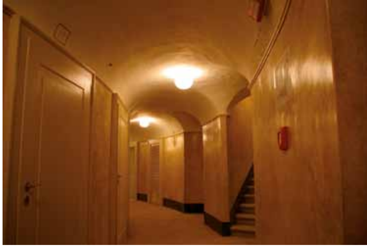
Fig. 5. The corridors and the new doors of the boxes after the restoration.
