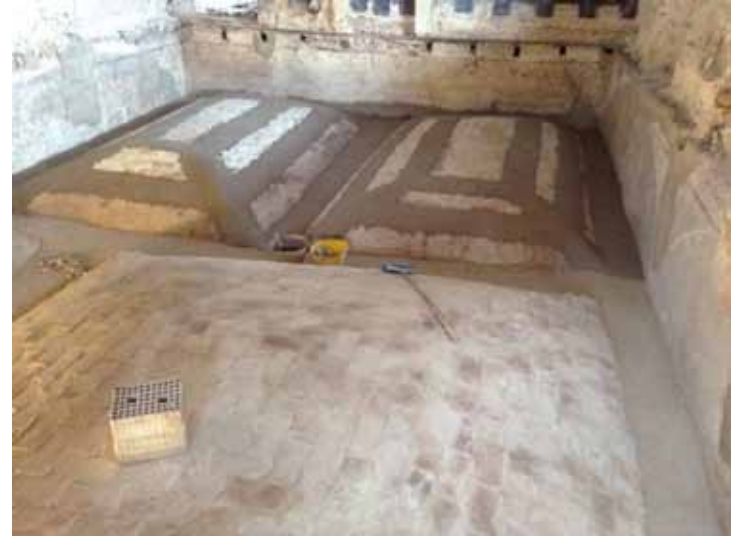
Fig.4. Consolidation of vaults by CFRP reinforcements.
