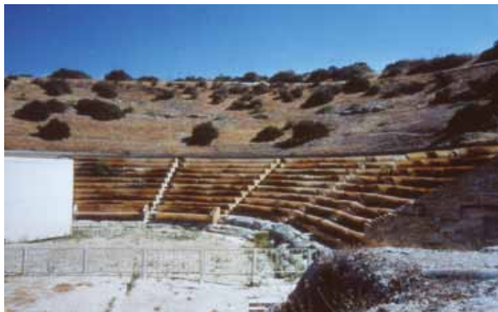
Fig. 1. Roof of the cavea of the Heraclea Minoa amphitheatre.
