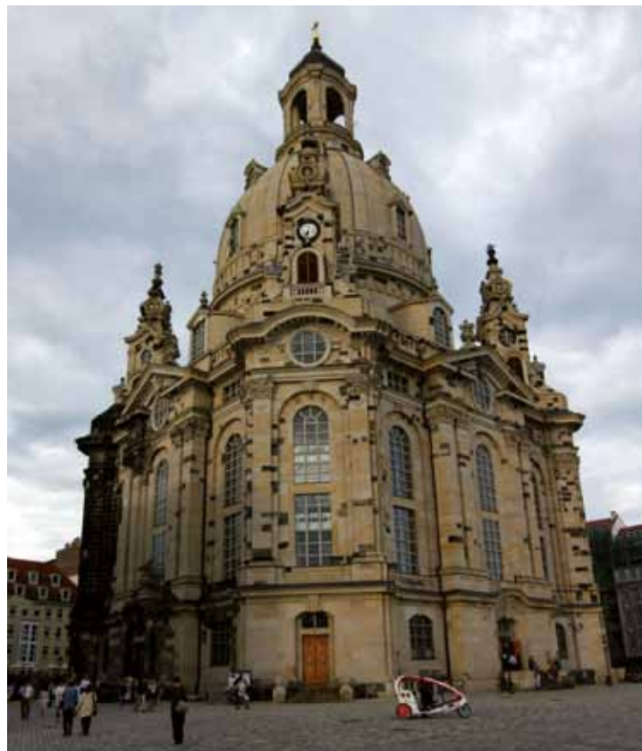
Fig. 3. Frauenkirche and Dresden: the reconstruction of the destroyed church with the integration of the missing parts and the original materials (1994-2005)
