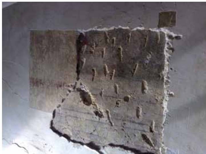
Fig. 5. Stratigraphic tests on decorated plaster.
