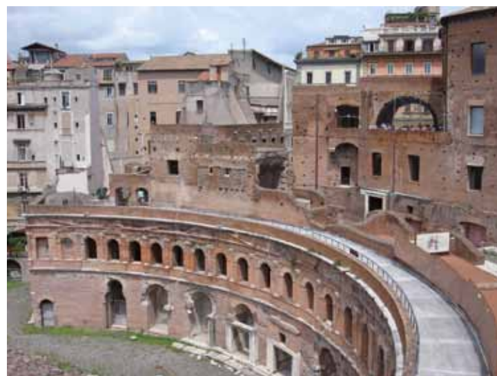
Fig. 2. Mercati di Traiano, Rome - General view of the Grande Emiciclo. The electrical systems for general and temporary displays in the "botteghe of Via Biberatica" were integrated into the new pavement.
