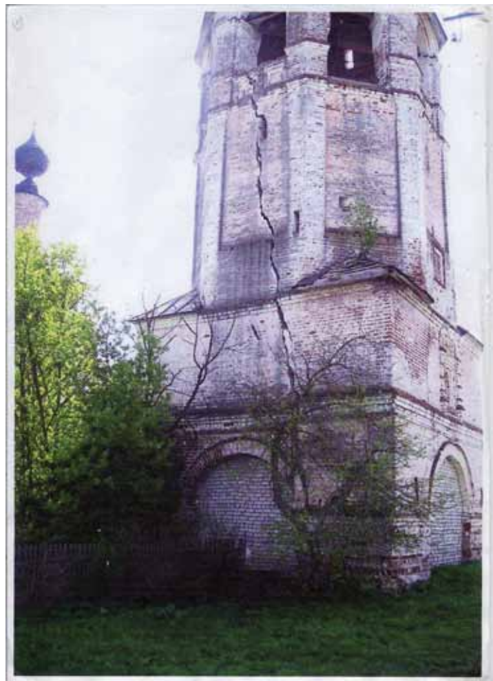
Fig. 2. Bell-tower's deformation.
