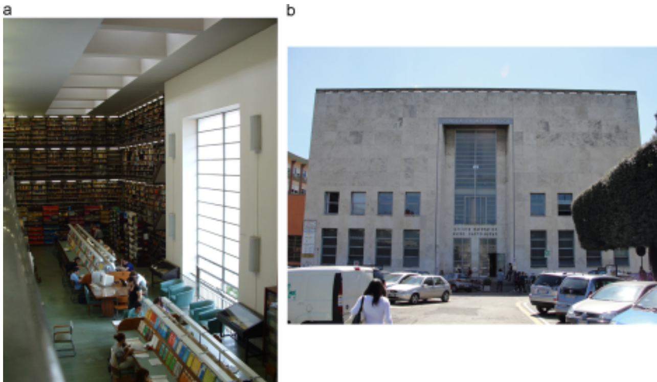
Figure 9 (a) The reading hall and (b) the front façade of the library today. The triple height has been reduced by cutting out the space at the lower level with a slab that is clearly visible from the street view (Salvo 2012).
