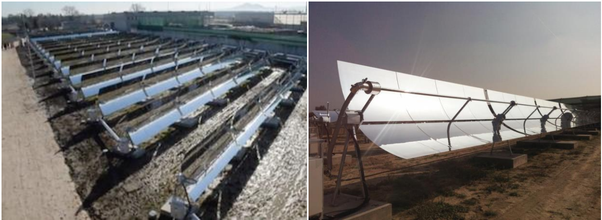
Figure 2 – Photo of the solar thermal plant and detail of a parabolic trough (right)
