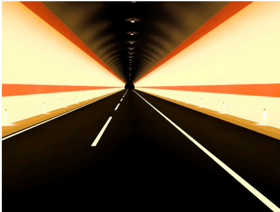
Figure 1. Rendering of the tunnel inner zone: backup lighting of the highway and lighting of the emergency exits along each side of the tunnel.
