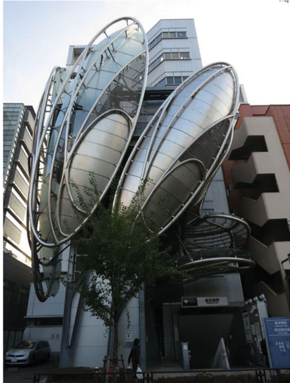
Fig. 86.6 Makoto Sei Watanabe. Iidabashi subway station, entrance at street level. The steel is realized straight from the same data files and can be considered the next higher level of generation. Photo: Courtesy Andrew I-kang Li
