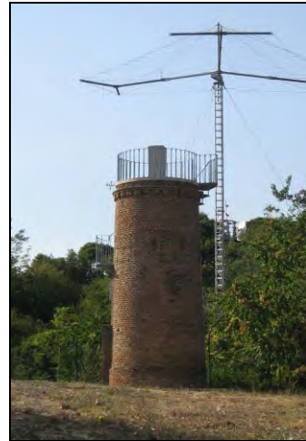
Fig. 3 The tower of Monte Mario, fundamental point of the old and the 1940 Monte Mario datum (photo of G. Timár)
