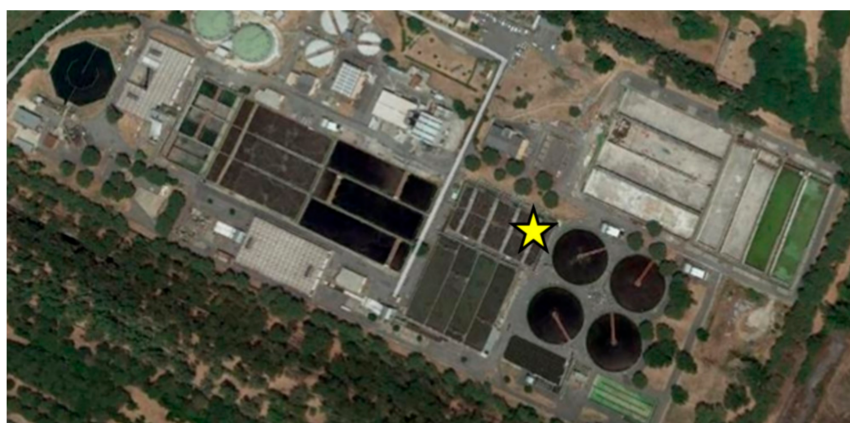
Figure 1. Wastewater treatment plants with the oxidation aeration tanks highlighted by the yellow star.
