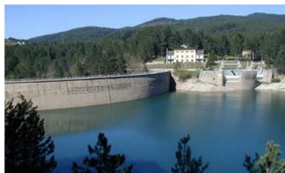
Figure 5. Cecita dam (source: https://www.enelgreenpower.com/ ; accessed on 20 January 2024).
