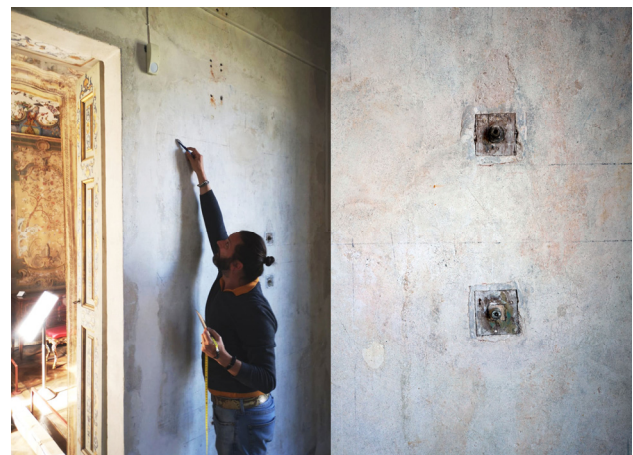
Figure 9. Identification of the geometric pattern for assembling the furniture and iron clasps in the cabinet of Villa della Regina (Photo: E. Pupi).
