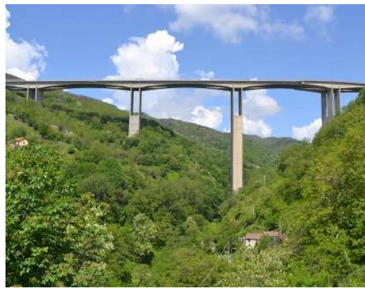
Figure 10. “Viadotto Gorsexio” with a central pillar taller than 172 m.
