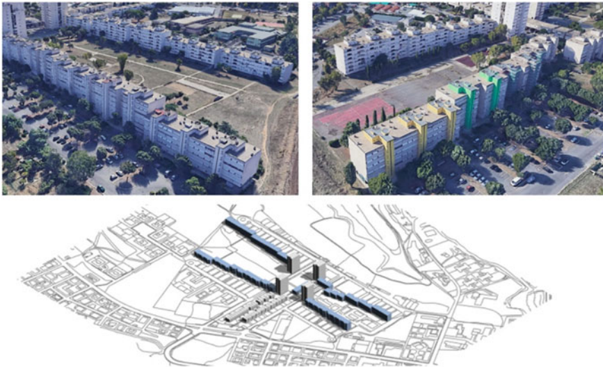
Fig. 5 The low-rise housing buildings
