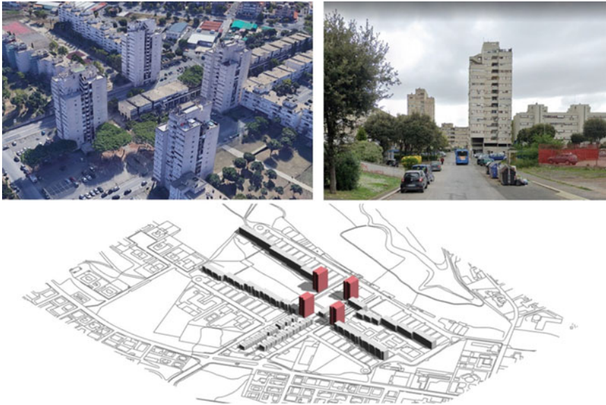
Fig. 6 The tower buildings
