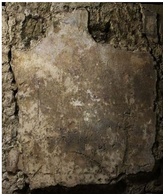
Figure 10. Orthomosaic of the graffiti-covered portion of the wall in Santa Sabina.
