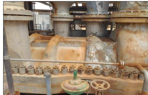
Fig. 1. Actual photo of the Centrifugal Compressor of the DP-STAH base
