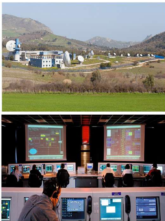
Figure 11.1. The Telespazio ground station at Scanzano (PA), Sicily (top), and its mission control room (bottom). The facility hosts multiple large-aperture parabolic antennas dedicated to satellite tracking, telemetry, and high-frequency communication. Its elevated location above Piana degli Albanesi provides low radio-frequency interference and an unobstructed horizon over the central Mediterranean, supporting both geodetic applications and operational satellite links. The control room enables real-time monitoring and coordination of atmospheric modeling, delay correction, and satellite link management.
