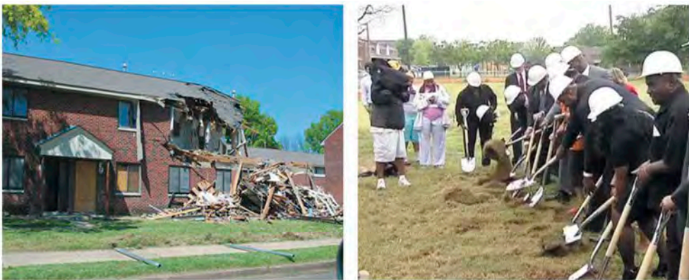
Figure 2. Demolition of Cleaborn Homes (on the left); Inauguration ceremony for the redevelopment of Cleaborn Point at Heritage Landing (on the right). Sources: Picture from the Memphis Flyer News Blog available at http://www.memphisflyer.com/NewsBlog/archives/2011/04/12/demolition-begins-at-cleaborn-homes and screenshot from news coverage available at https://www.youtube.com/watch?v=ZzbU3ukfAcQ .
