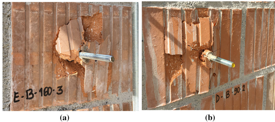
Fig. 7 Combined sliding failure and block cone failure (a) and combined sliding failure and block failure (b)
